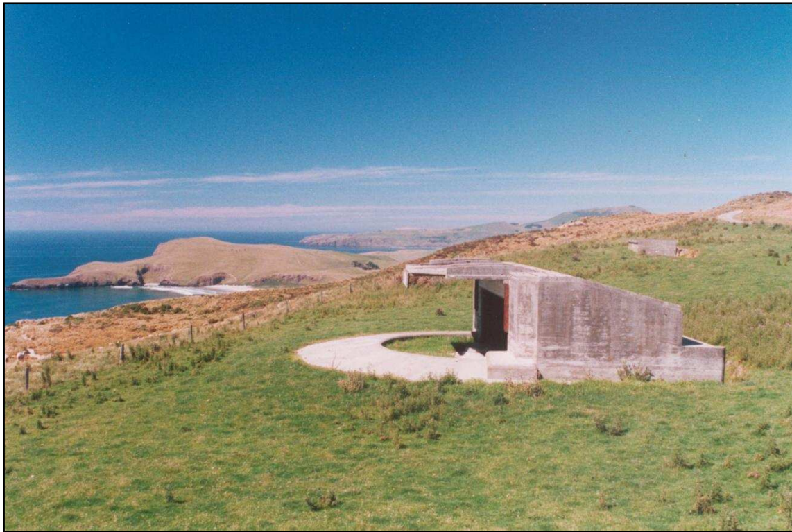
Figure 20. 6-inch gun emplacement at Rerewahine Battery. Second emplacement is visible in background. c. 1985. Condition of structures now is reportedly poor (Photo courtesy of Laurie Stewart, Otago Peninsula Trust).
