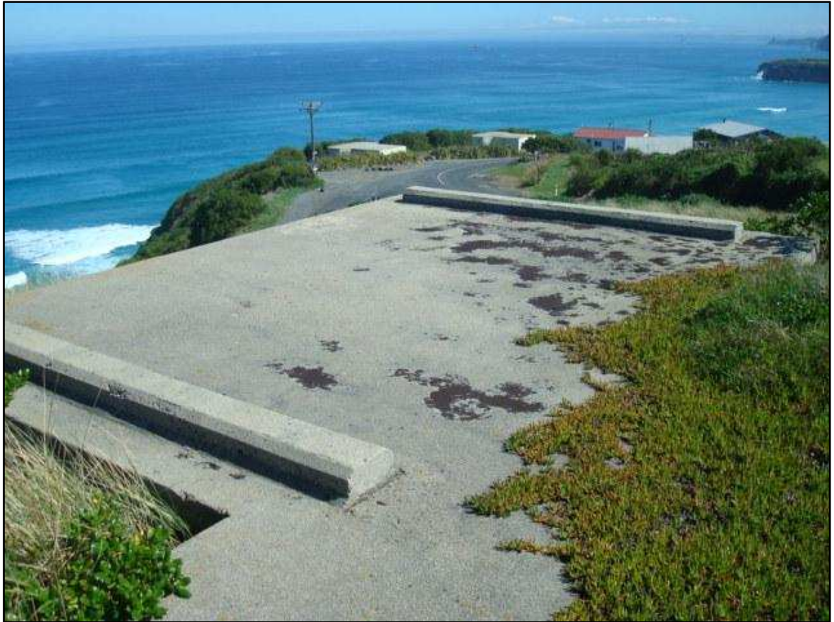
Figure 19. Partially exposed roof of Observation Post at Tomahawk Battery. The two 6-inch emplacements are visible in the top centre of photo.
