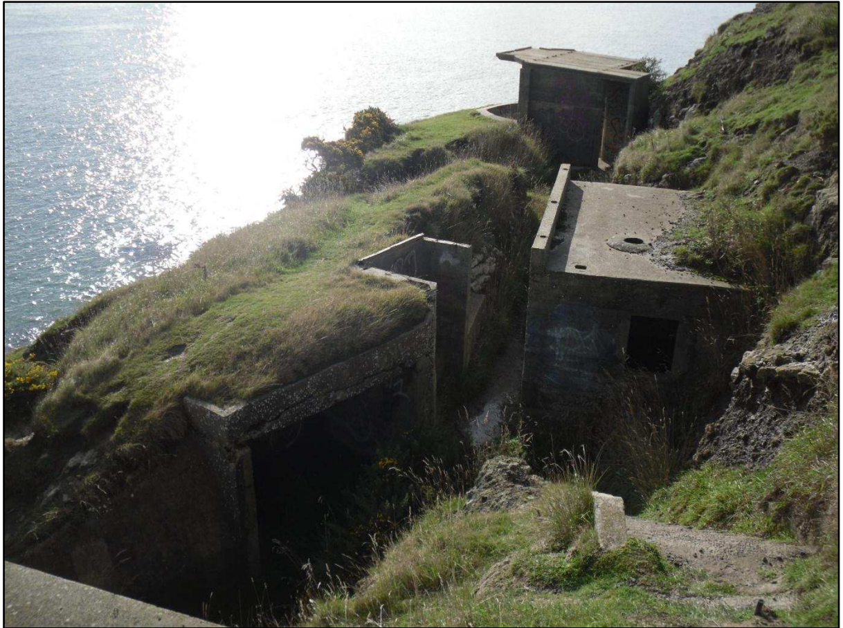
Figure 16. Harington Point lower level. Northern QF gun emplacement is visible in background, while corner of southern QF emplacement is visible in bottom left corner of photo. The war shelter is visible in between the two QF emplacements.
