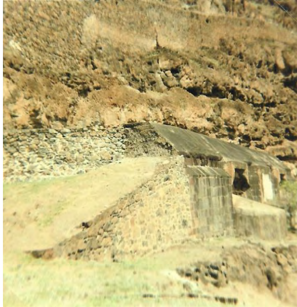
Plate 5: Munden's Battery, casemate type for 3 guns Built c. 1880. The original battery was built here in 1673.
