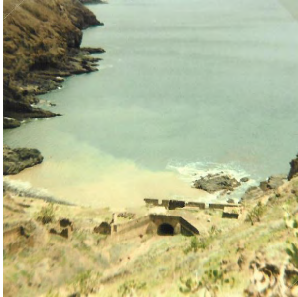
Plate 14: The ruins of Banks Platform, with only about one third of the original curtain wall remaining.
