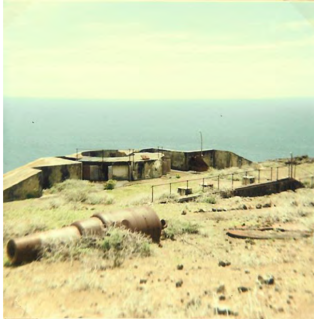
Plate 9: Munden's Hill East Battery with old gun nearby dated 1872, but it was not mounted in this Battery which had a later type pedestal mounted gun in its circular platform.
