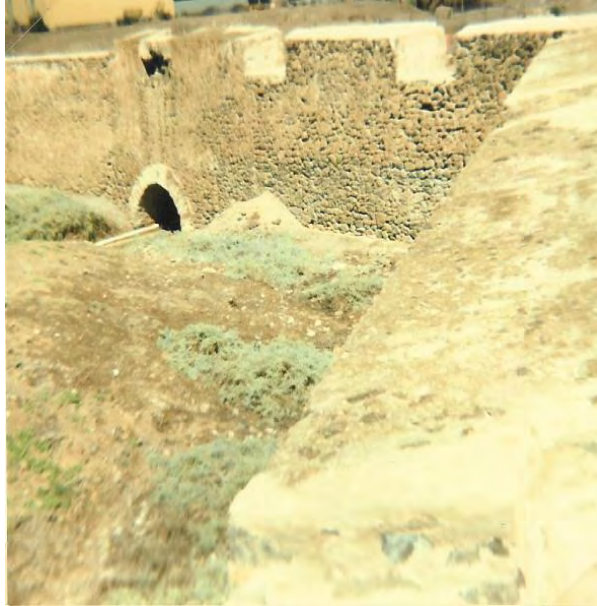
Plate 23: Rupert's Line curtain wall with storm water tunnel that had a portcullis.
