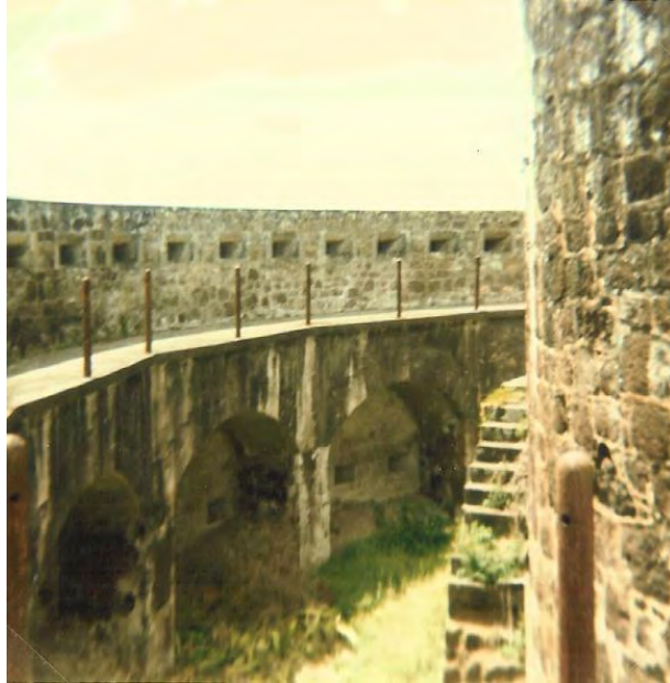
Plate 40: Loopholed platform at High Knoll Fort Steps up the side enter the tower, and gave access to gun platforms above.
