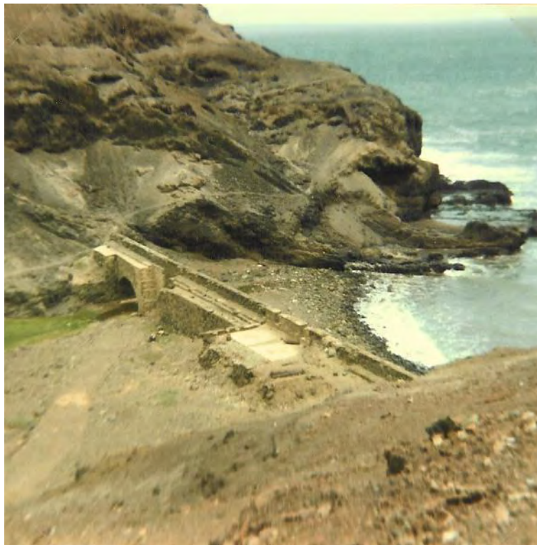
Plate 28: Inland view of Sandy Bay Line eastern side, flanked by Crown Point. The gun platforms are at centre.
