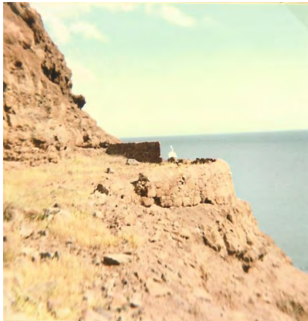
Plate 3: Patton's Battery, cut into cliffs above West Rocks Built during the term of Governor Patton (1802-07) as a redoubt for James Line.
