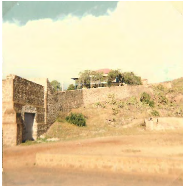
Plate 44: Ladder Hill Fort. Perimeter wall loopholed for musketry defence. Behind the wall is Red Roof House.
