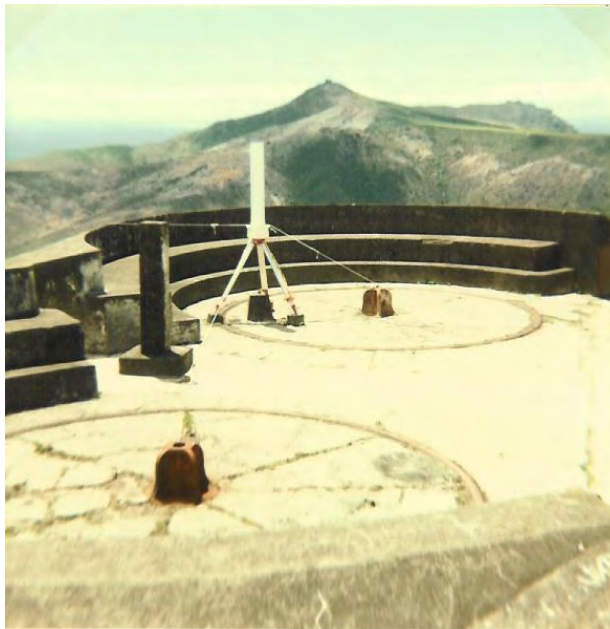
Plate 41: Gun platforms on top of High Knoll Fort with Flagstaff Hill in the distance. Pivot points and traversing tracks for guns are shown.
